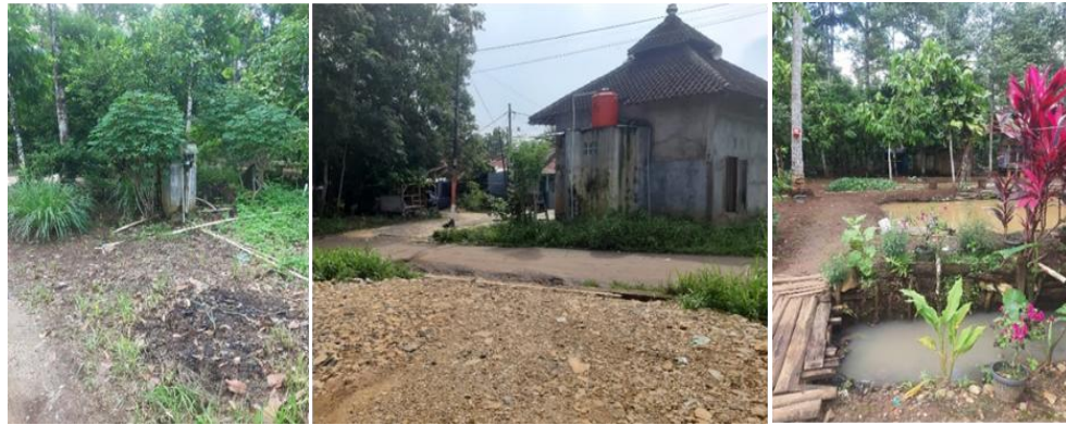
Figure 3. Evaluation of highland water control to reservoirs in Gedong Tataan Village
